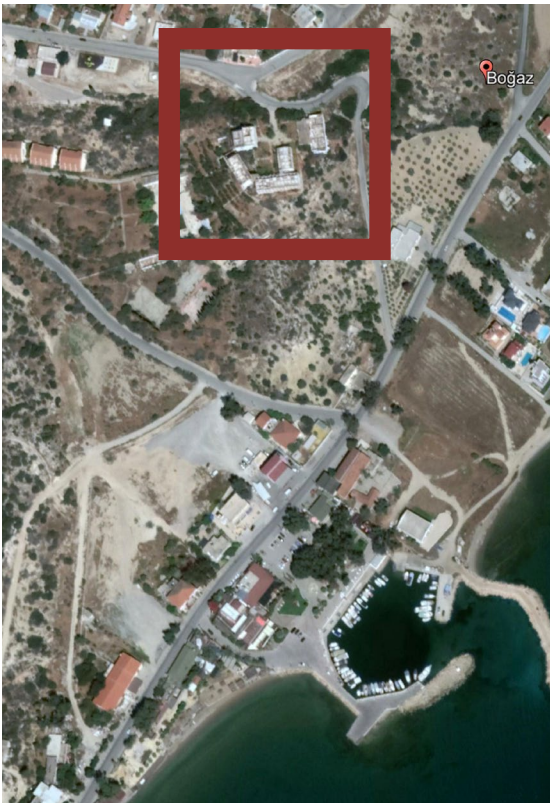
2018, Google Earth Images Removed Roof Tiles & Structure
